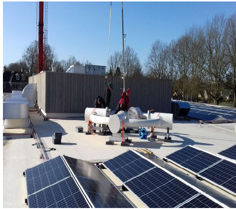
Figure 1.8: Installation of the roof top thermoacoustic chiller
